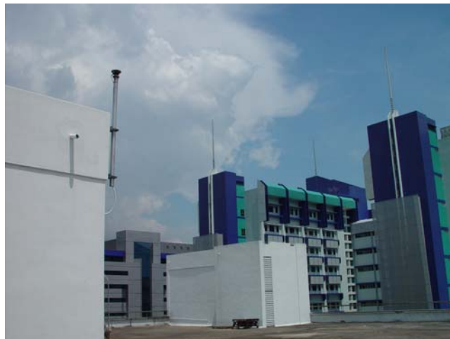
Figure 4 Base station antenna
